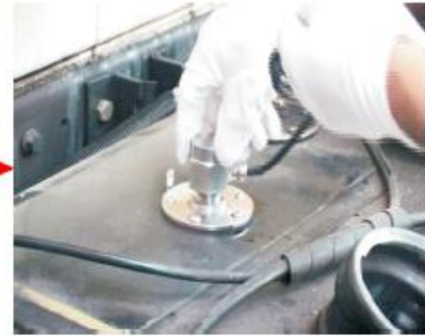
9. Installing the sensor
