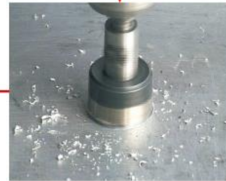
8. Drilling hole on the tank
