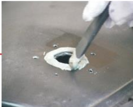
7. Smearing Sealing Material
